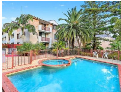
21/1 Hume Avenue Castle Hill
