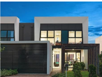
18 Messenger Street Kellyville
